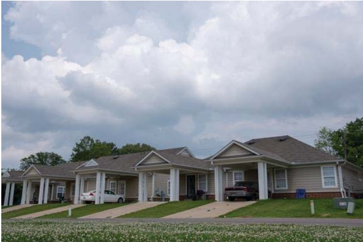
Unity Lane crosses through rows of quality affordable housing. (Brandon Dahlberg)
